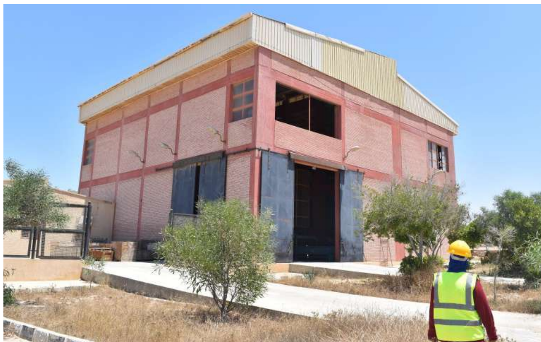
Figure 17: Fluorescent Lamps Processing Facility at Nasreya Hazardous Waste Landfill
